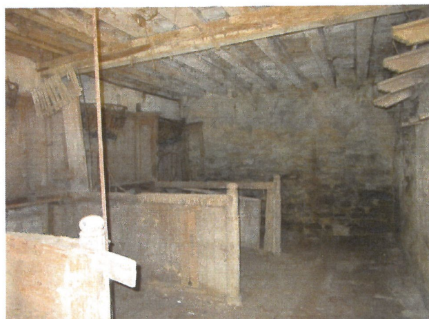
Stall (EG / Scheune)
